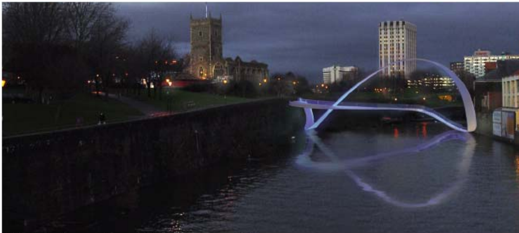
↑ The deck, arch and pier are one and the same, which gives the structure an economy and lightness.
