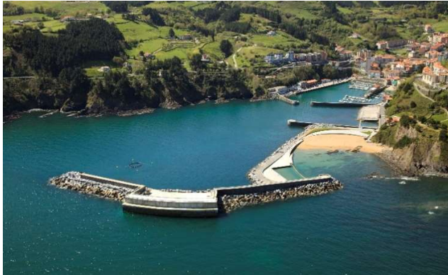
Fig. 1. Wave Power Plant of Mutriku in Spain.
