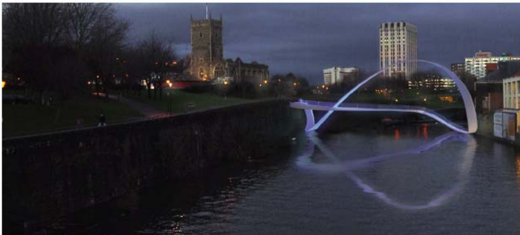
↑ The deck, arch and pier are one and the same, which gives the structure an economy and lightness.
