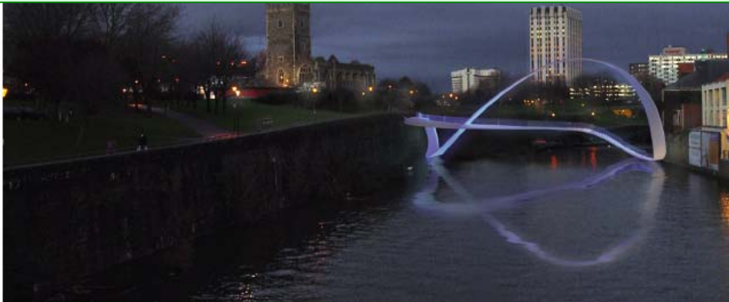
↑ The deck, arch and pier are one and the same, which gives the structure an economy and lightness.
