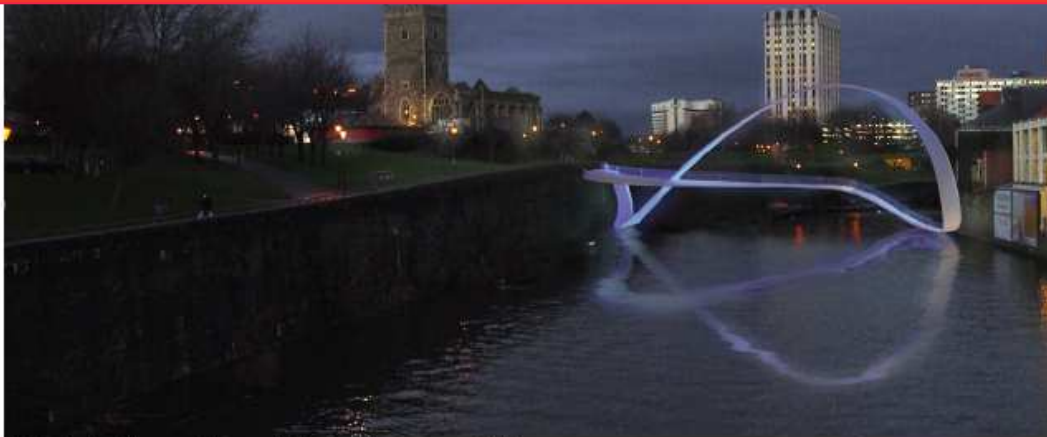
↑ The deck, arch and pier are one and the same, which gives the structure an economy and lightness.
